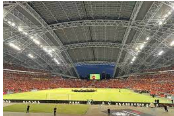
National Stadium- Singapore
